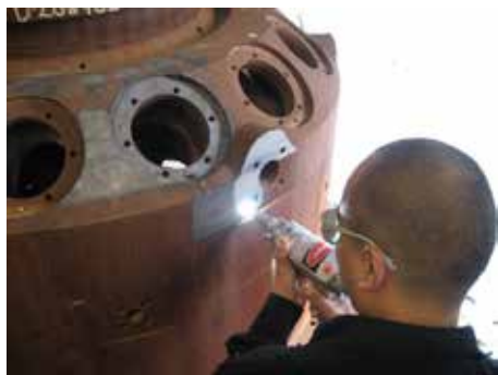
Rust removal (image courtesy General Lasertronics)
