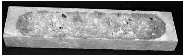
A laser scabbled surface. The block is 100 mm wide and 300mm long. Beam diameter was 80 mm and a 5kW Nd:YAG laser at TWI Cambridge was employed.
